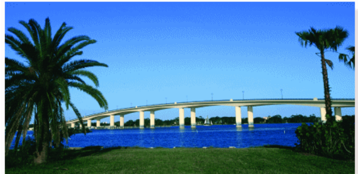
Broadway Bridge, Daytona Beach, FL – Versiflex™ Elastomeric Bearings
