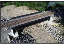
through-girder bridge supported on precast concrete abutment seats and 5'-0" diameter drilled shafts. The design accommodated construction of drilled shaft foundations outside the footprint of the existing bridge to allow for continuous rail operations up until the scheduled track outage.
