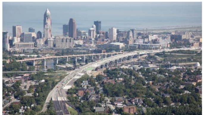
Eastbound George V Voinovich Bridge
