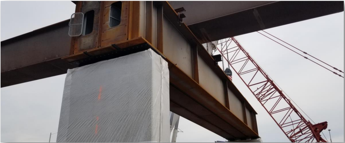
Tub Girder Erected
