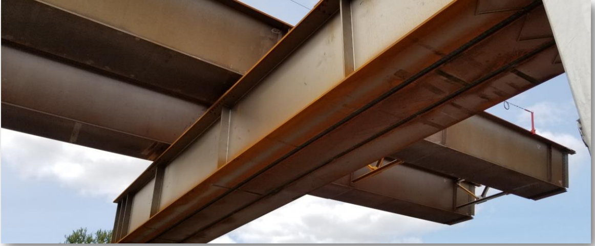
Second Tub Girder Erected
