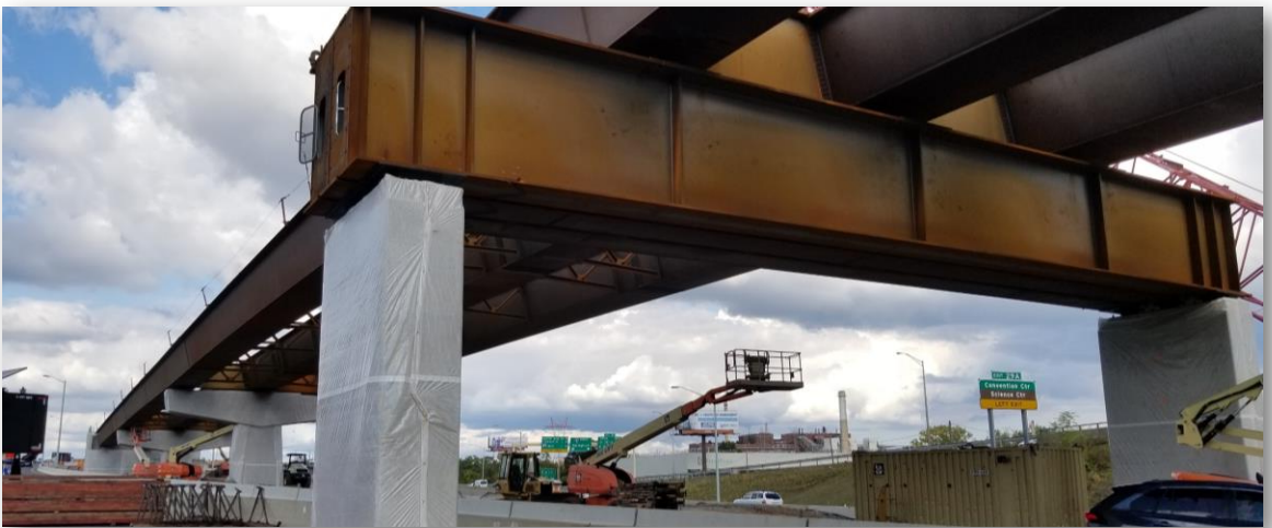
Erection of all Spans Complete
